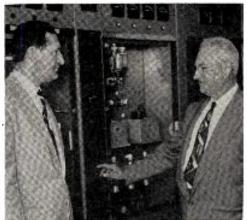
WSMB New Orleans executives John R. O'Meallie (I), vice president-general manager, and Harold Nebe, chief engineer, prepare to throw the switch on the station's new 5 kw RCA transmitter. WSMB is undergoing an engineering overhaul, and now has a 5kw standby transmitter and a 35 kw standby generator.
